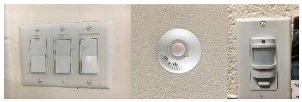
Figure 14 - Wall Switches and Occupancy Sensors
