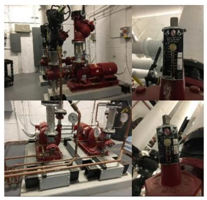
Figure 17 - Hot Water Pumps and Motors and Partially Opened Triple Duty Valves
