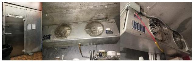
Figure 30 - Walk-In Refrigeration Equipment
