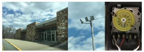
Figure 15 - Exterior Lighting and Timeclock Control
